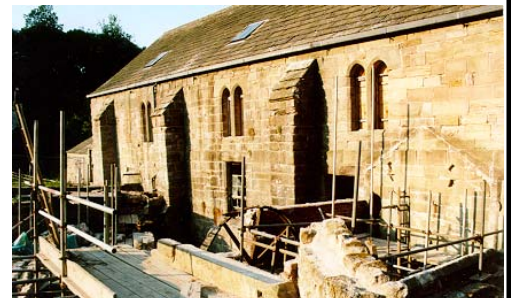
The Mill during restoration work.
